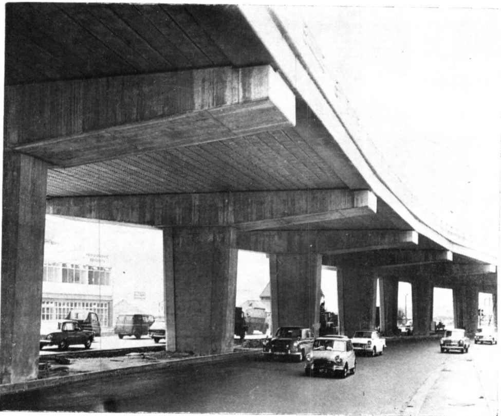
Fig. 4. Elevated motorway on natural rubber bridge bearings
