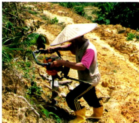
(b) A mechanical digger (soil borer) is used at sloping areas
