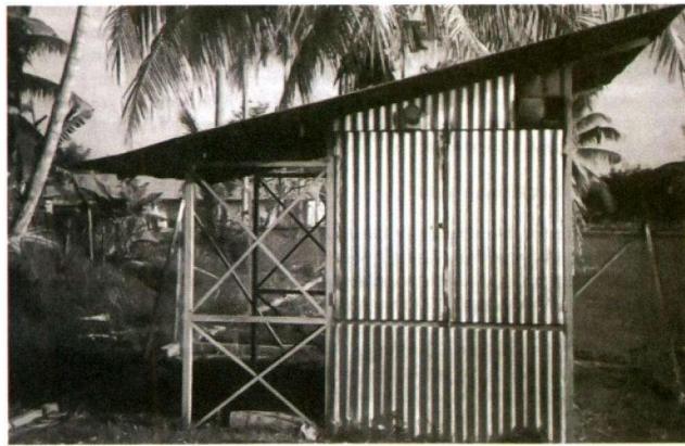
(b) RRIM aluminium-walled smoke cabinet
