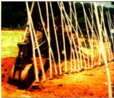
(c) Extracting core stumps with the help of an excavator at bud-break stage
