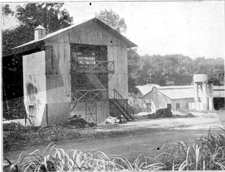
GENERAL VIEW OF DOUBLE "DEVON" SMOKE-HOUSE AND FACTORY BUILDINGS.
